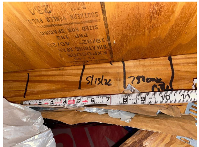
Field=6 Inch Deck Fastener Spacing
